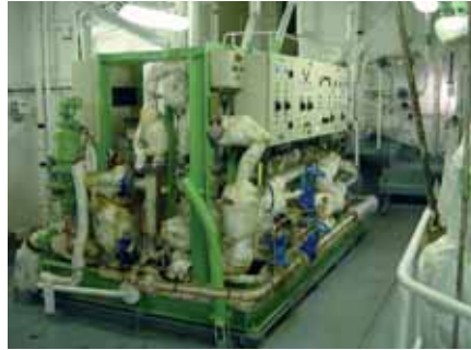
Design for a modular solution – Ready-mounted, on-board fuel block
